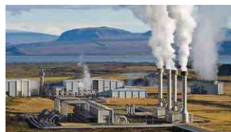
Fig 8.11(b) Geothermal power plant
