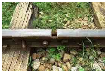
Fig 9.13 Gaps between Rail Tracks
